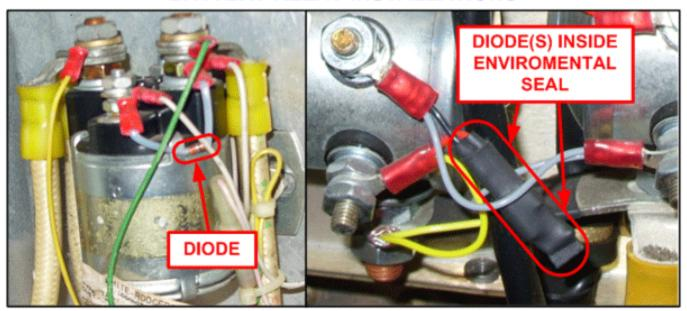
A diode is connected across the input wires of inductive loads, such as relays, to protect voltage sensitive avionics, electrical components and switches. The diode (known as a "Fly-Back Diode") is reverse-biased. When the circuit is energized, no current flows through the diode. However, with the current flowing through the inductive load there is a magnetic field which provides power to the relay motor, or valve.
